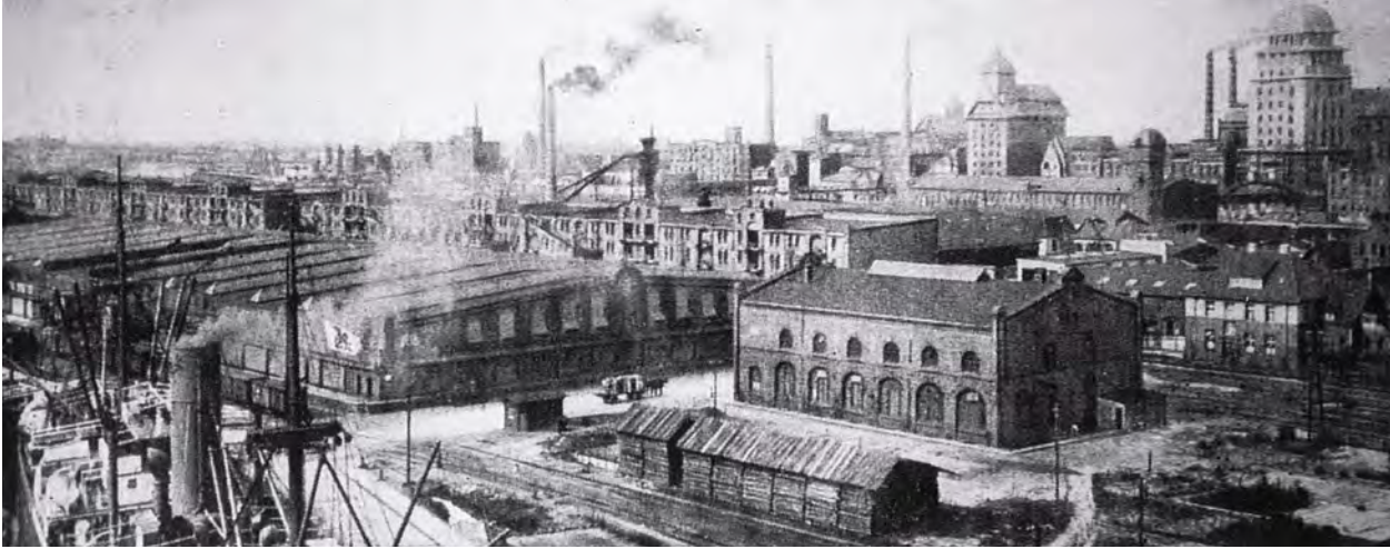
Power control center and Shed 13 prior to World War II
