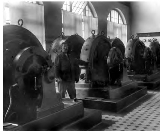
Transformer in the power control center
